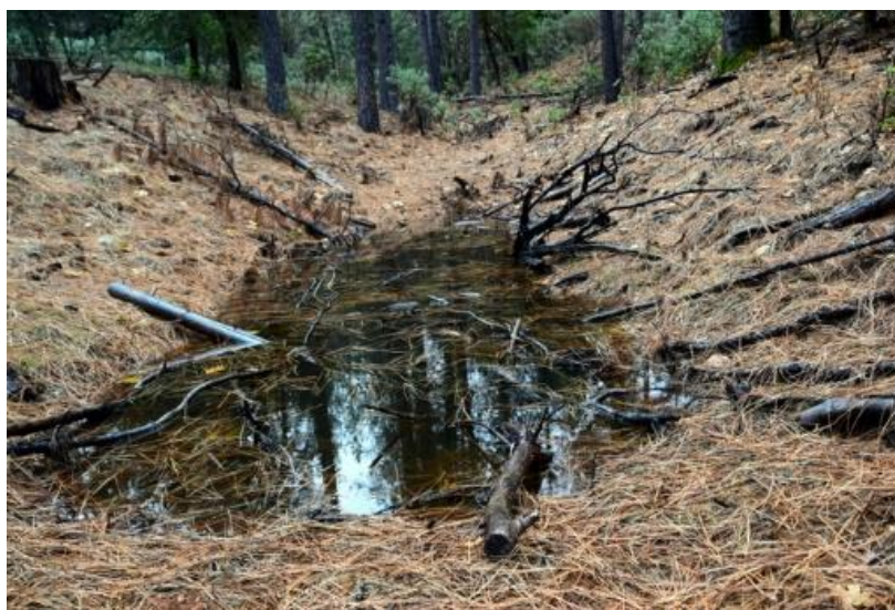
This small wetland was built on higher ground in only one-half day near a tributary to Bear Creek on the Eldorado National Forest in 2014.
