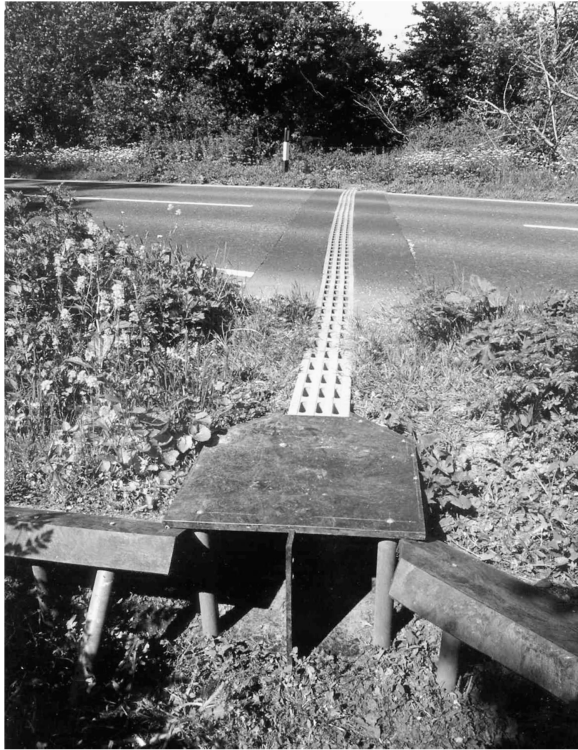
Figure 4. Toad tunnel at Newhaven, UK. Reproduced with permission of ACO Polymer Products.
